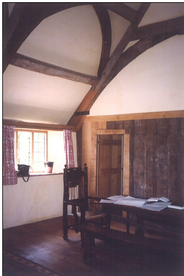
The repaired screen in its new position.
