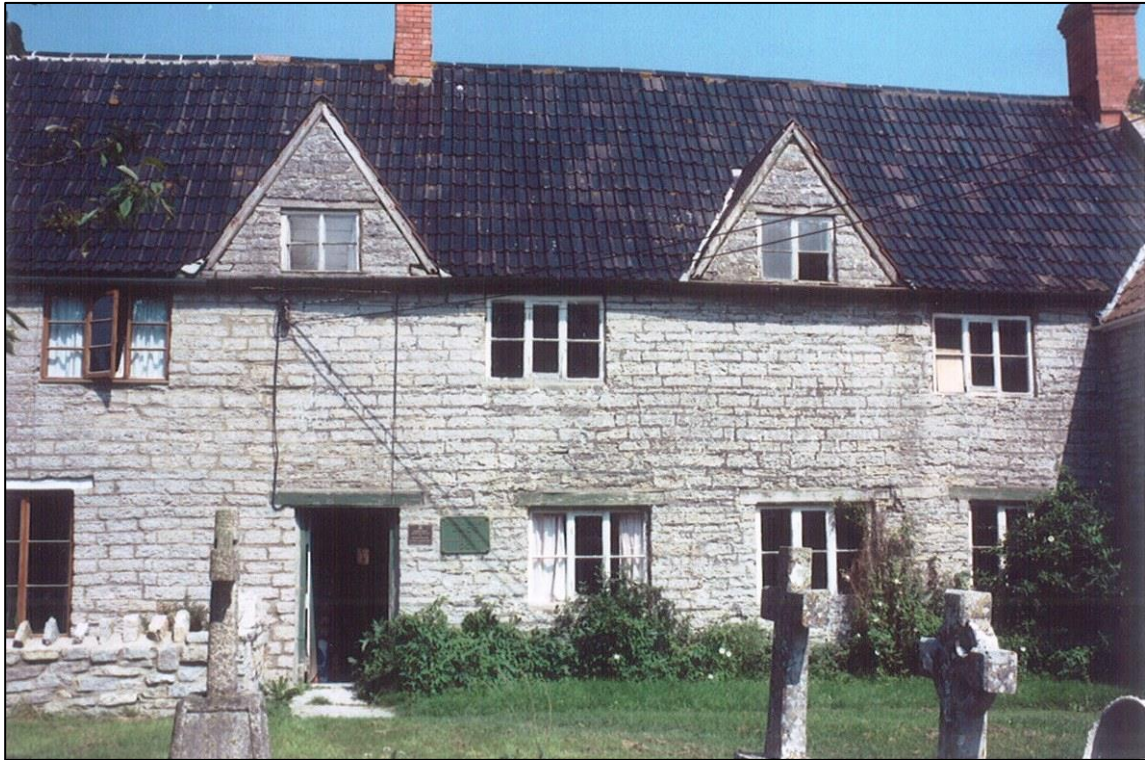
The wirescape was removed and placed underground.
