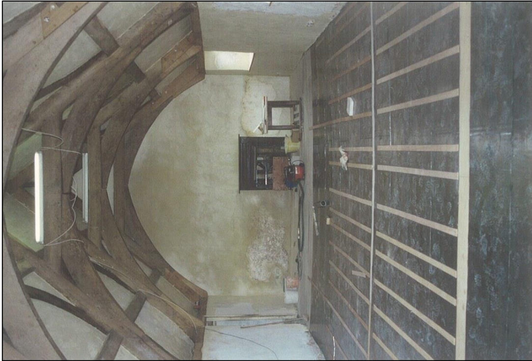
Looking east before the partition went in. The fire surround was removed.
