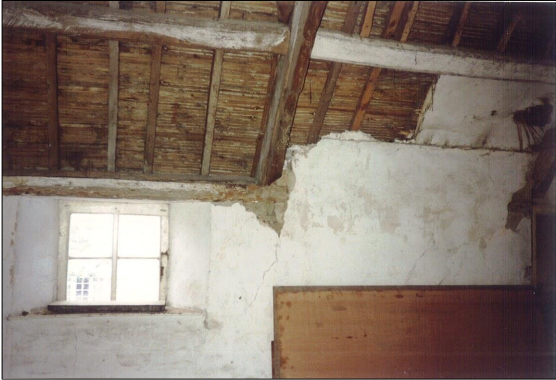
The old west facing window in the kitchen previously hidden by the lean-to.
