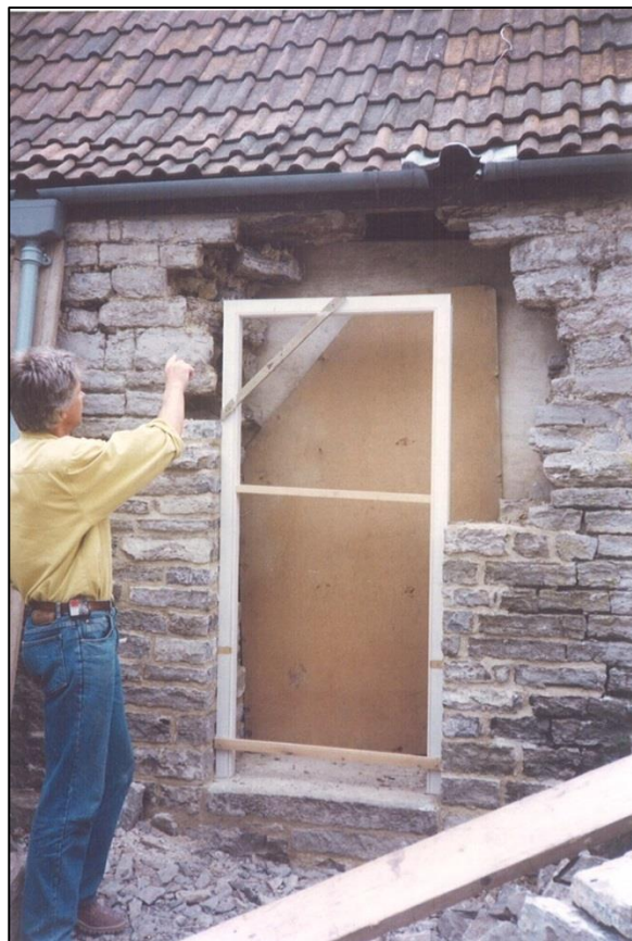
Len Hardy trying out the new door frame.
