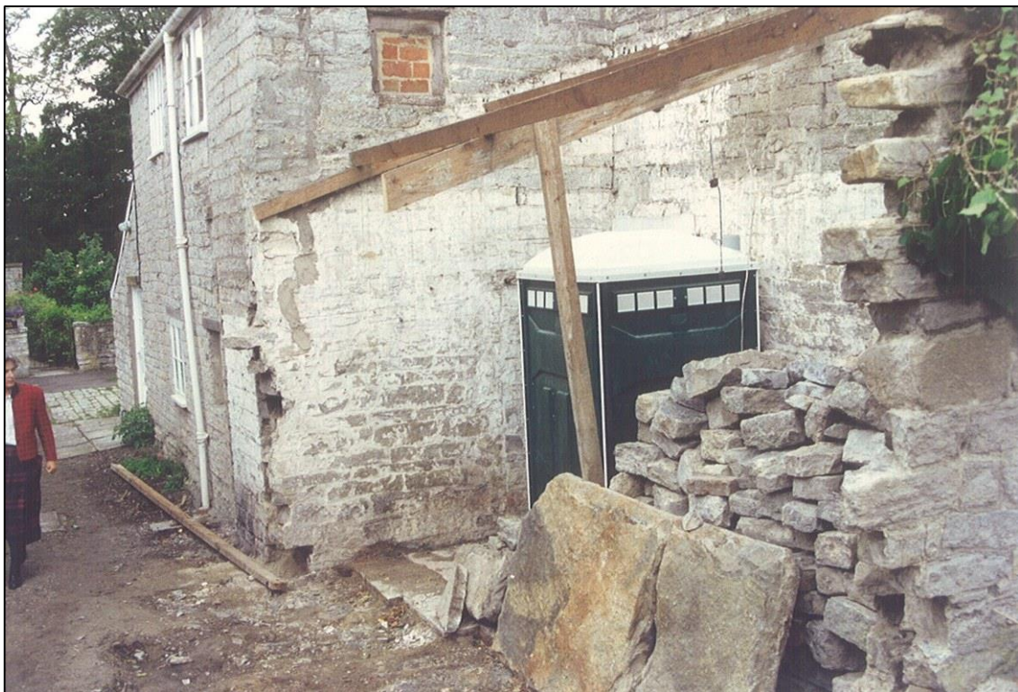
The lean-tos were demolished. Note the blocked up early window.
