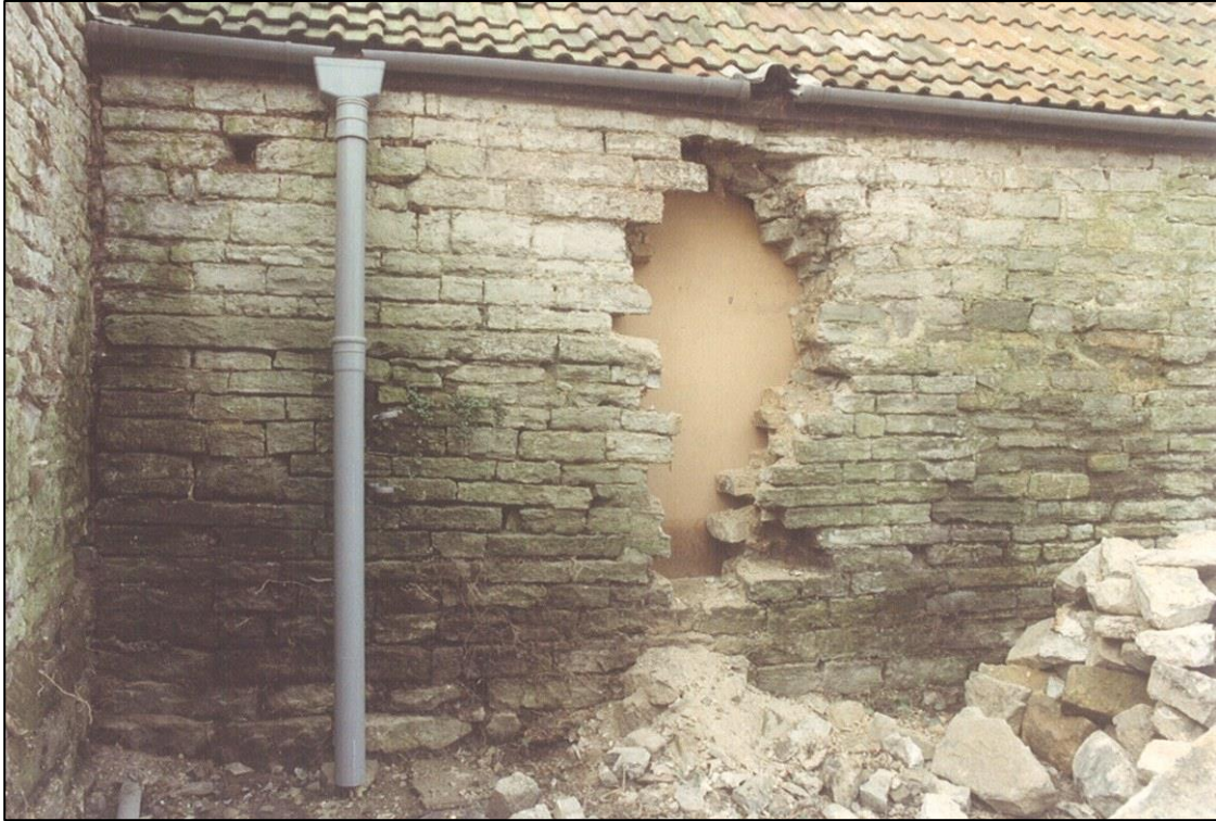
The opening for the front door.
