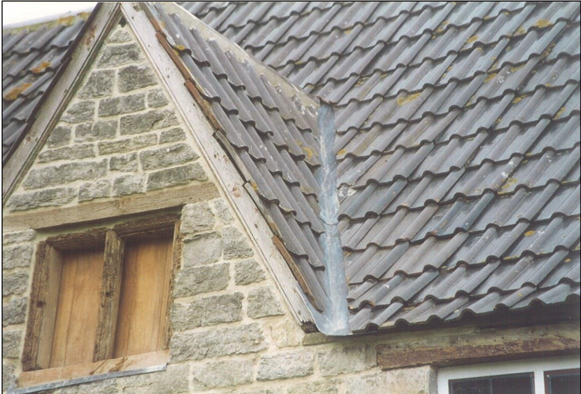
The attic windows were repaired and then boarded up.
