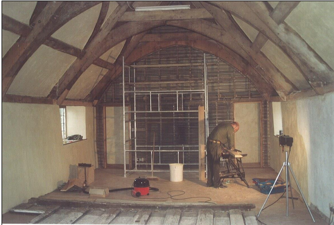
The 17th-century screen on the floor being repaired.
